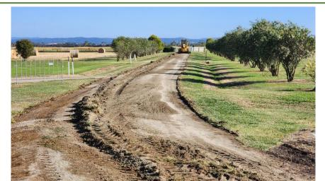
Starting work on profiling the driveway, with Glenn's big grader making easy work of it.
