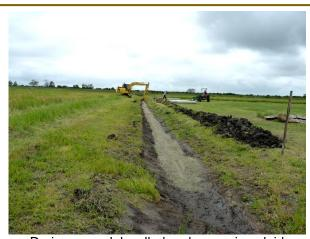
Drain scoured, levelled and screenings laid
