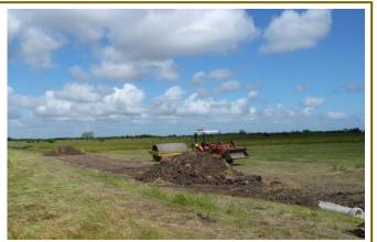
Filling almost finished, now requiring topsoil and final levelling, + sprinkler addition, at a later date
