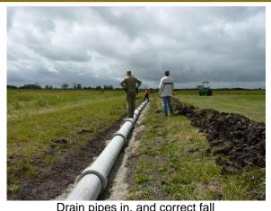
Drain pipes in, and correct fall
